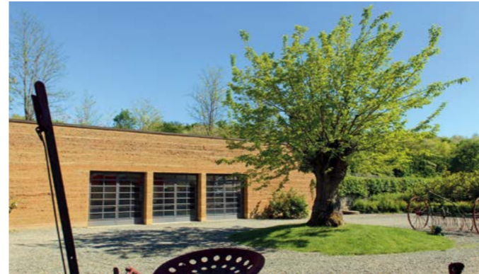
La Raia's wine cellar with its pisé (raw soil) wall made by Martin Rauch (© C. Dutton)
