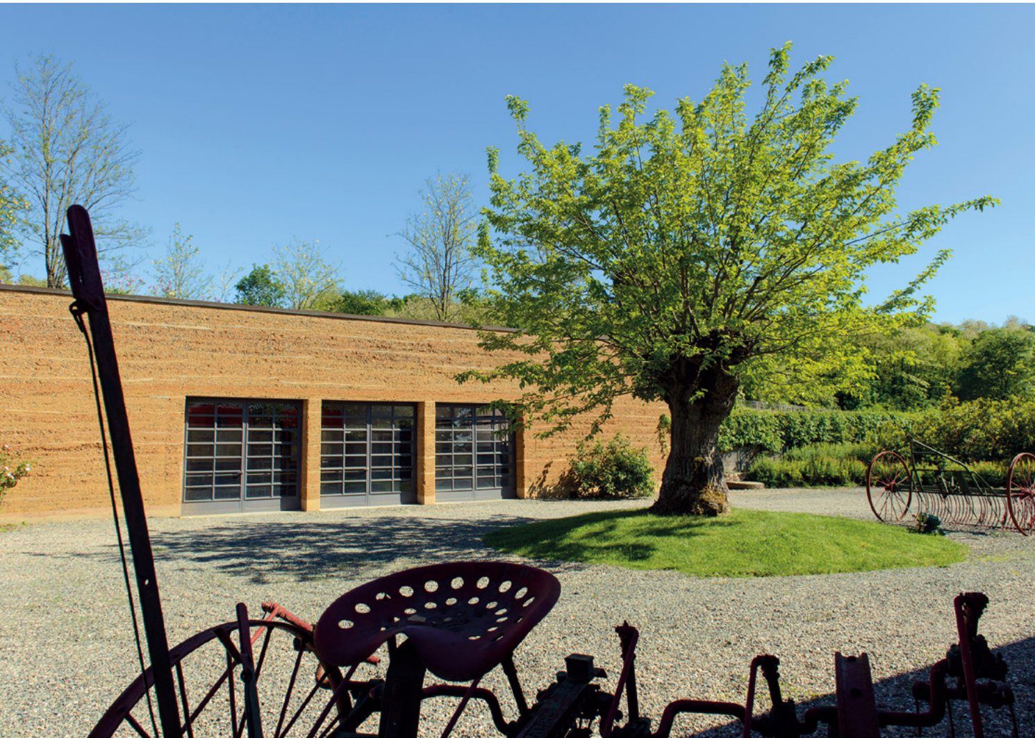
La Raia winery with its pisé (rammed earth) wall by Martin Rauch (© Colin Dutton)
